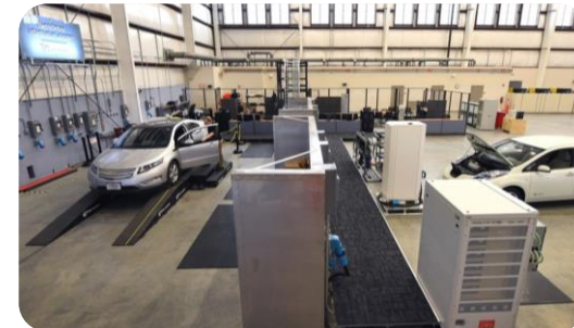
Electric Vehicle Infrastructure Laboratory (EVIL)
